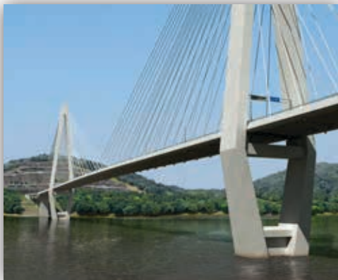
The new Ironton Russell Bridge.
