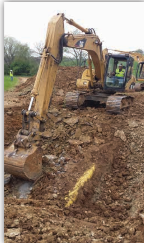
Contractors Rental on the pipeline job in Carlisle, KY
