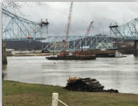
The old Ironton Russell Bridge coming down.
